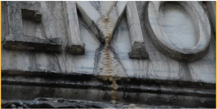
The Monument is literally crumbling due to decades of water damage.
