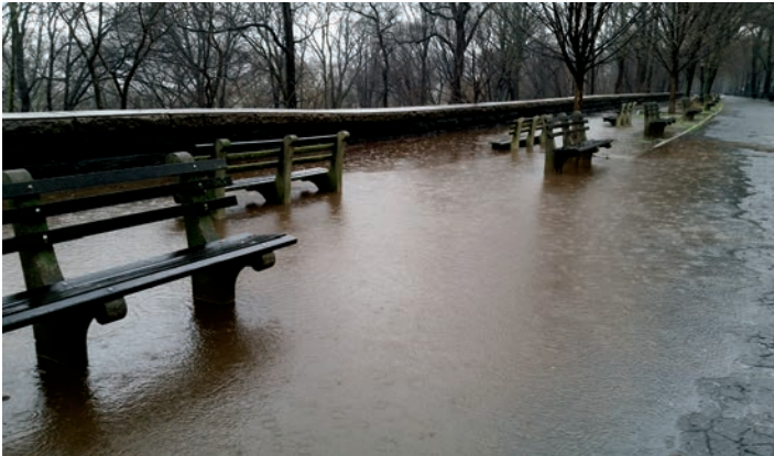
The aged drainage infrastructure inhibits the Park from absorbing and filtering rain water properly, which results in major pooling of stagnant water on paths.
