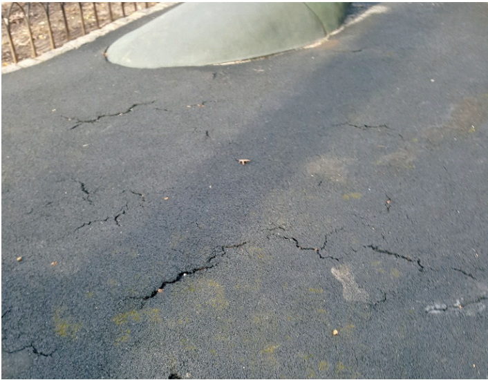
The pavement was cracked and damaged, presenting a potential safety hazard for children.
